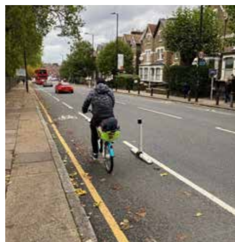
Light protected track with "wands"
