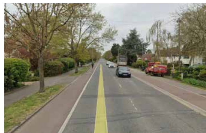
One-way (stepped) protected track (right) and on street cycle lane (left)
