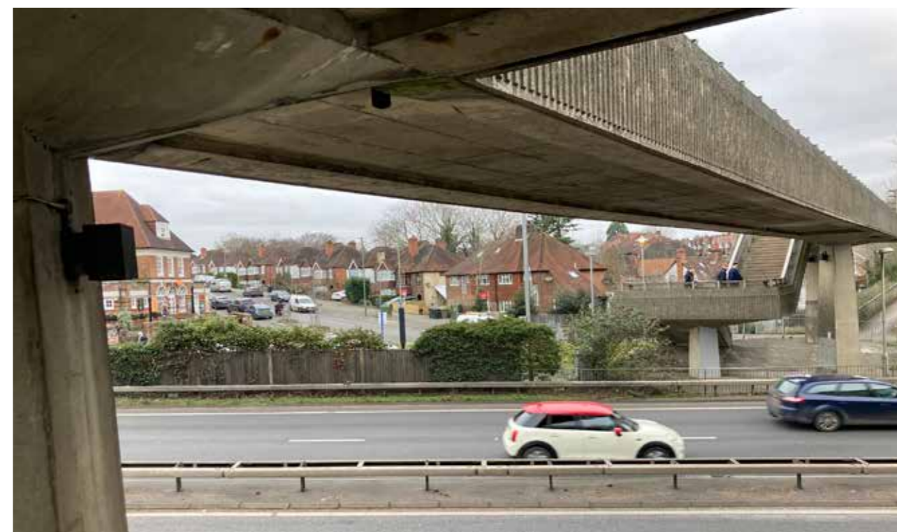
Figure 17 Pedestrian Bridge from Northwest of Guildford over the A3
